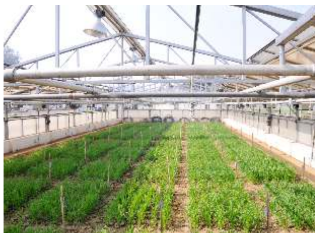
Fig. 1.5 Temperature controlled phenotyping facility
